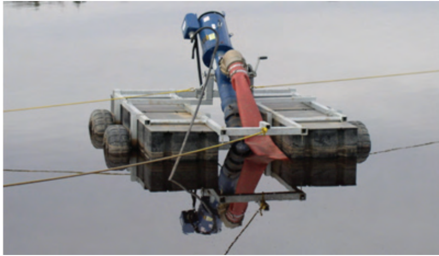
Figure 4. Floating pump installation for pumping lagoon water to a center pivot.
